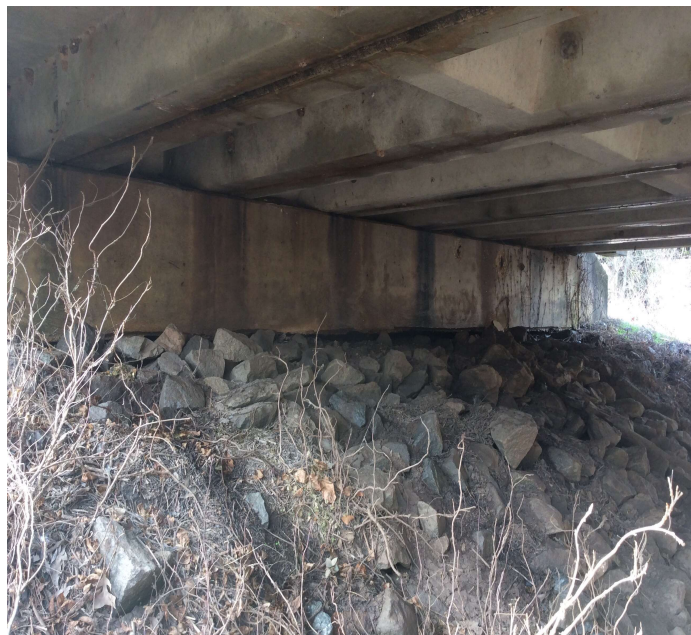
PHOTO 1 Description Endslope - Bent 1 (minor settlement)
