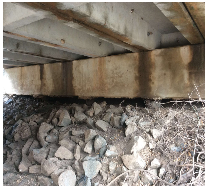
PHOTO 2 Description Endslope - Bent 5 (settlement)
