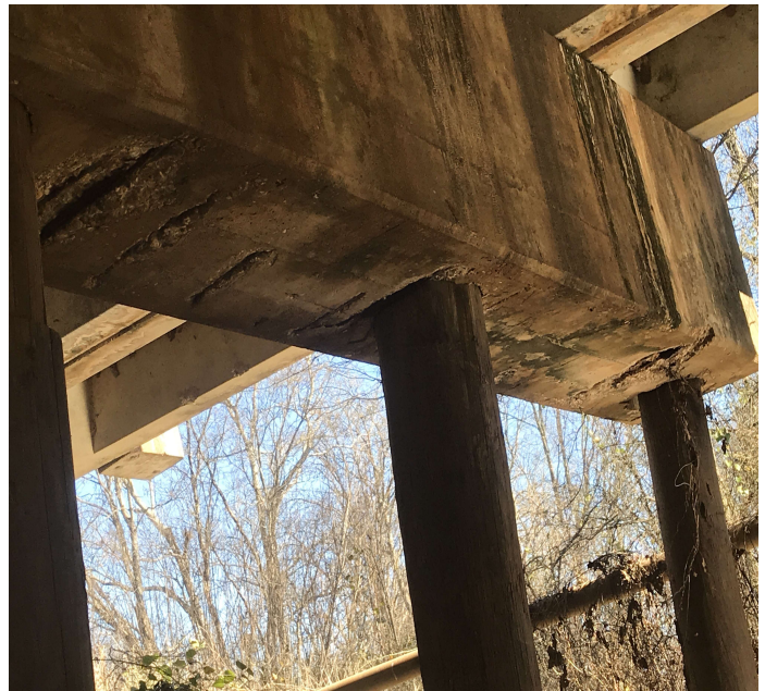
PHOTO 2 Description Bent 4 cap has spall with exposed rebar under and on edges of cap.
